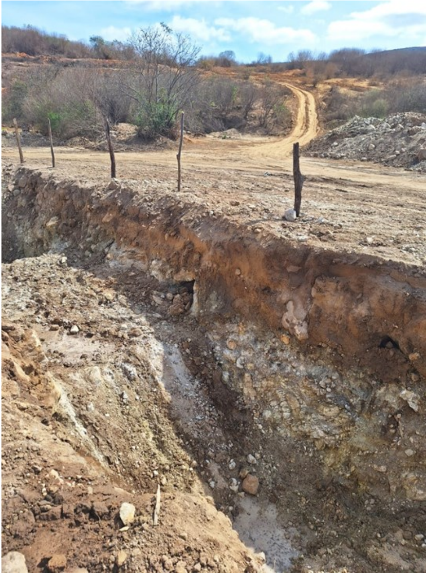
Figure 2: Trench in Anitta 2 showing lithium-bearing pegmatite at near-surface level
